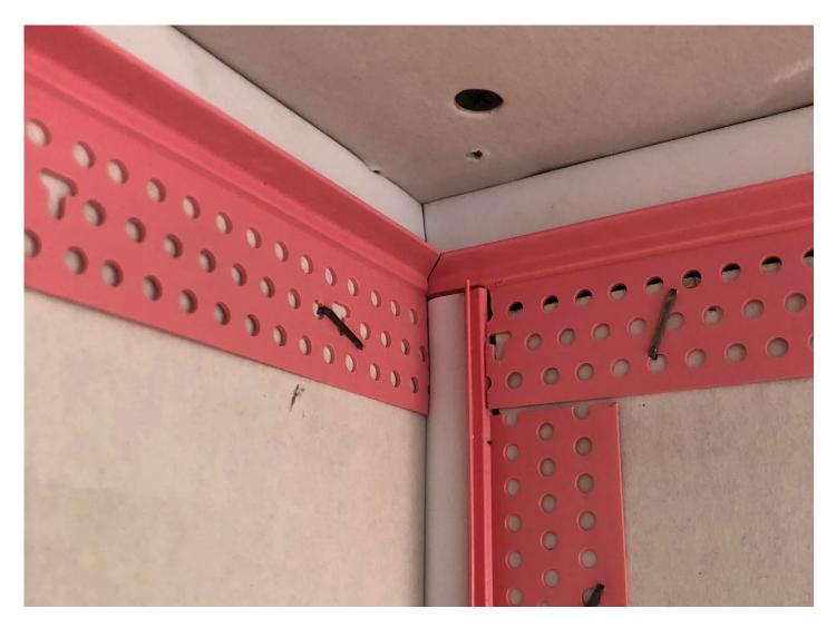
The outlier here is the Fire Rated 093V Expansion bead. This is used — specifically and exclusively — for control joints, where it eliminates the extra steps of applying fire rated
